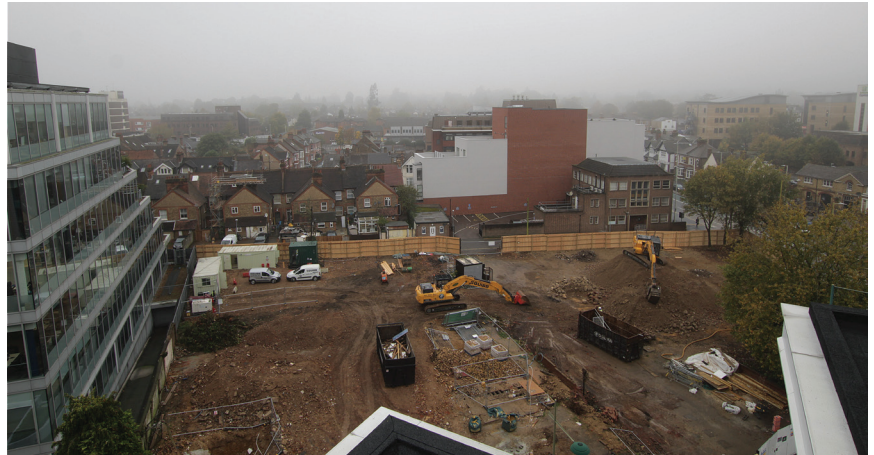
/ Cleared site as at 19 th October 2017
