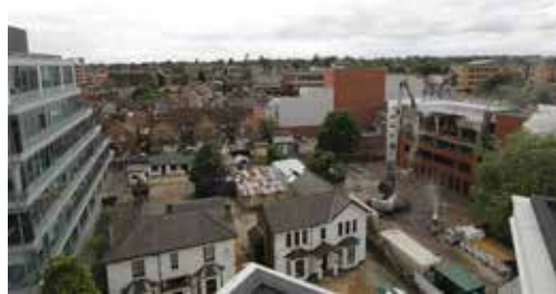
/ Demolition commencement on 3 August 2017
