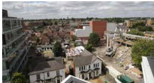
/ Demolition progress at 10 August 2017
