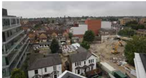
/ Demolition progress at 23 August 2017
