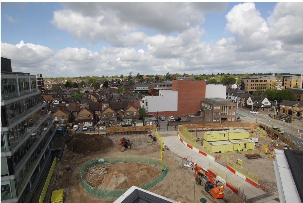
/ Cleared site from Clarendon Road, 25 April
