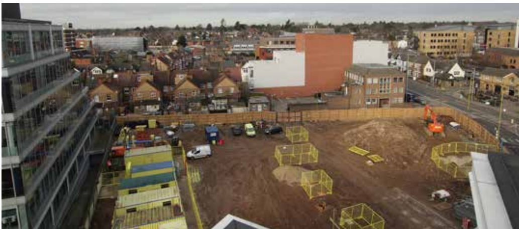
/ Cleared site from Clarendon Road, 5 February
