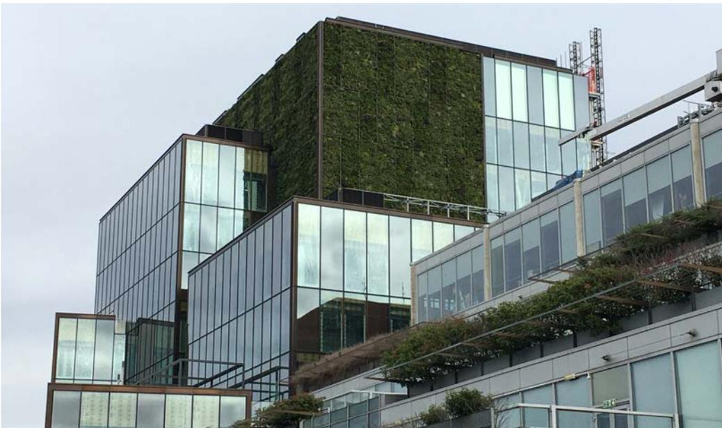
Photo showing the green wall, which is made of plants growing vertically on the side of the building.
